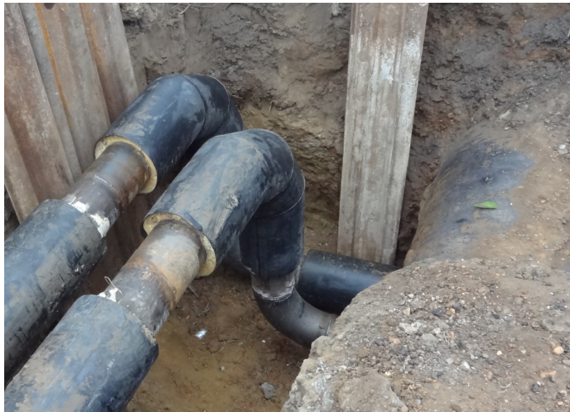
Fig 5 – On site solution for a hidden obstacle (1m dia unrecorded conduit from another DH Network)
